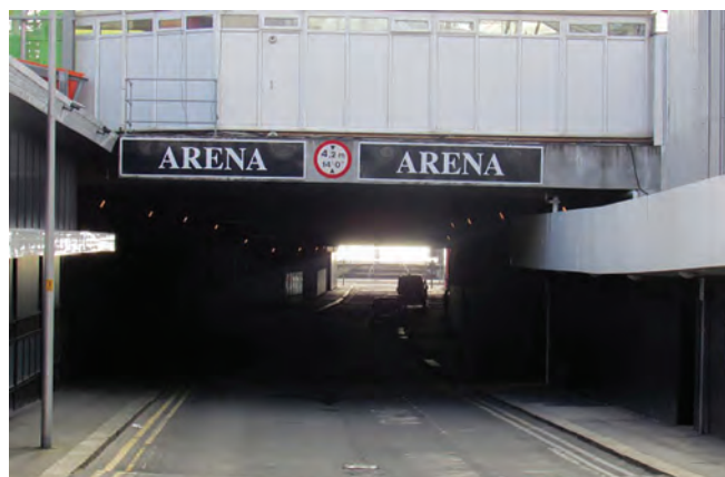
Tunnel under the Pleasure Beach on Watson Road, Blackpool, looking west
